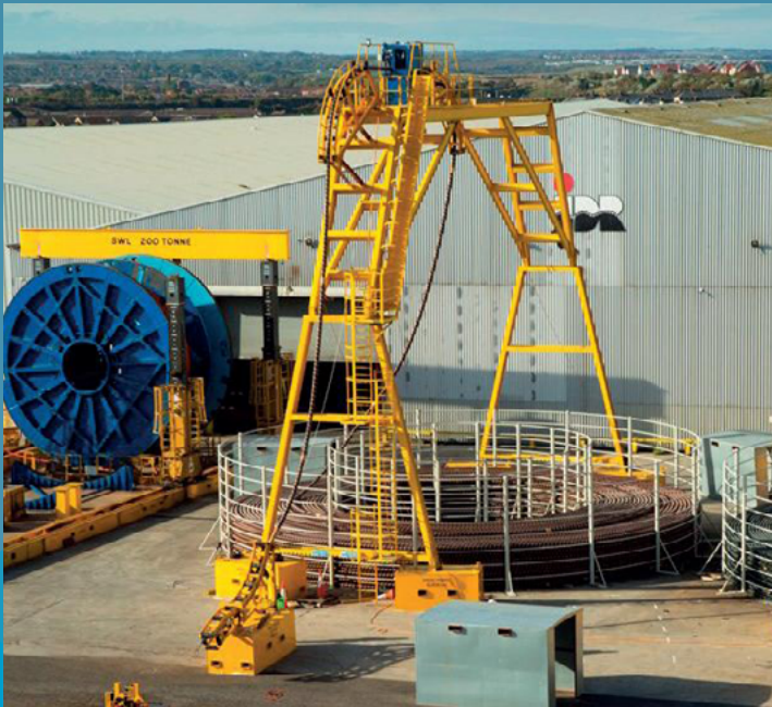
Cables being spooled for Moray East offshore wind farm. Image courtesy of JDR, all rights reserved.
